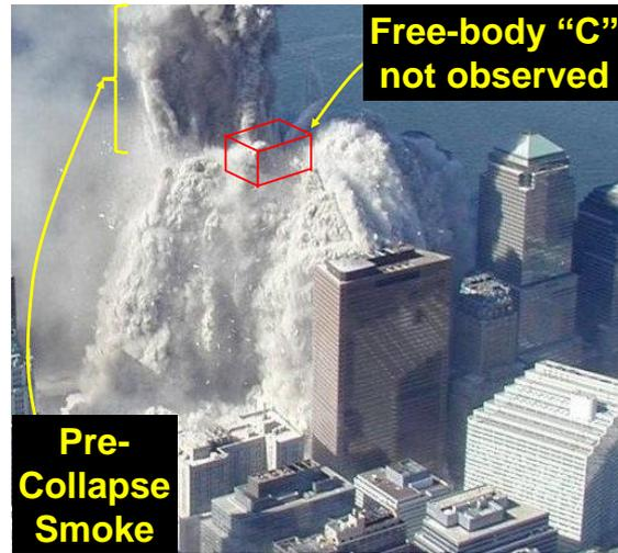
Fig. 2. Observation of Collapse Lacks Hypothesized Free-Body “C” (WTC1)
